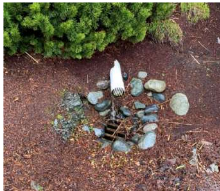
Figure 33. Dufferin Crescent, Nanaimo, parking lot stormwater runoff directed into a rain garden; however, it pours into a stormwater drain rather than the rain garden.
